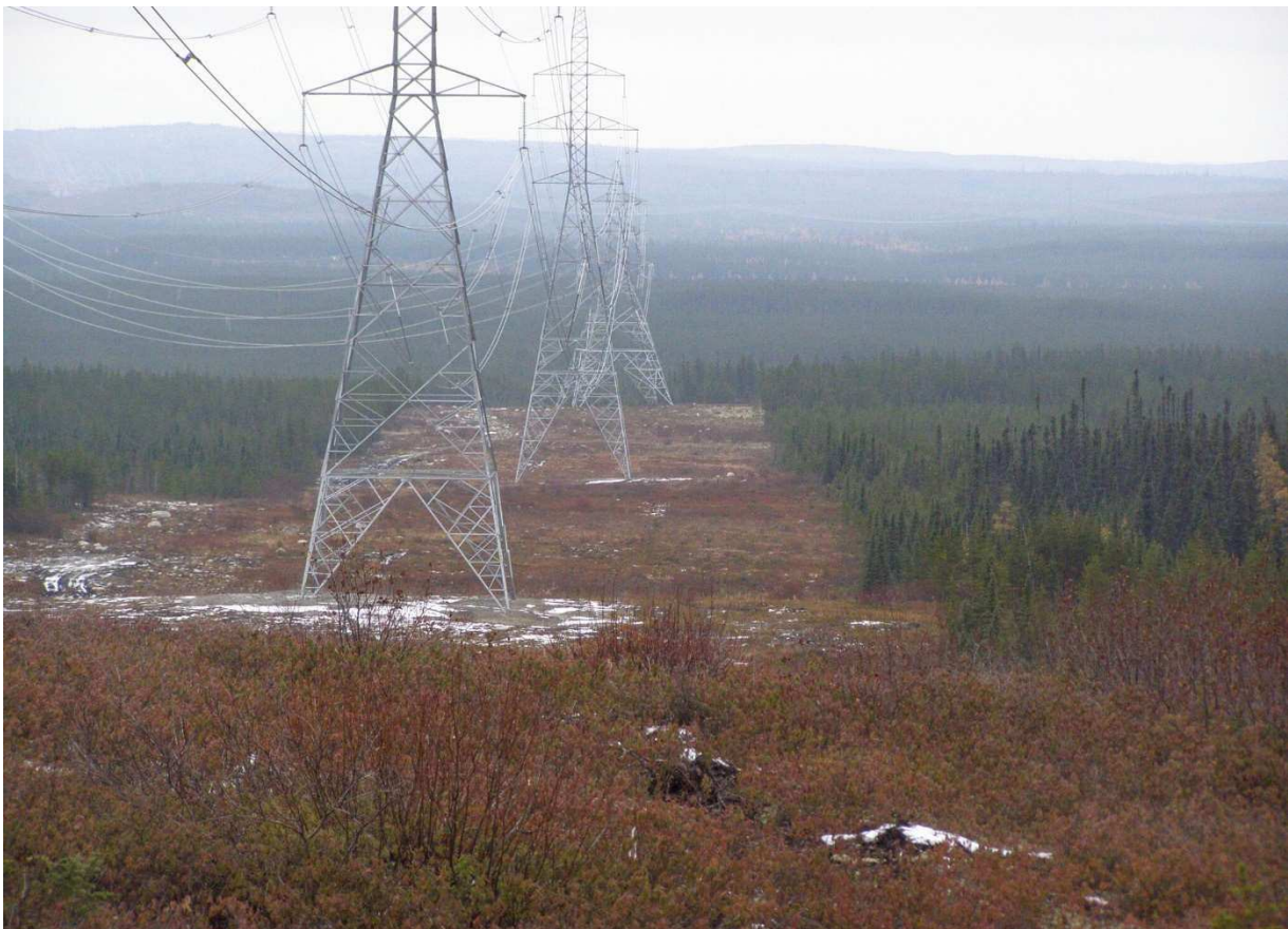
Power line at Rose Lithium-Tantalum site
