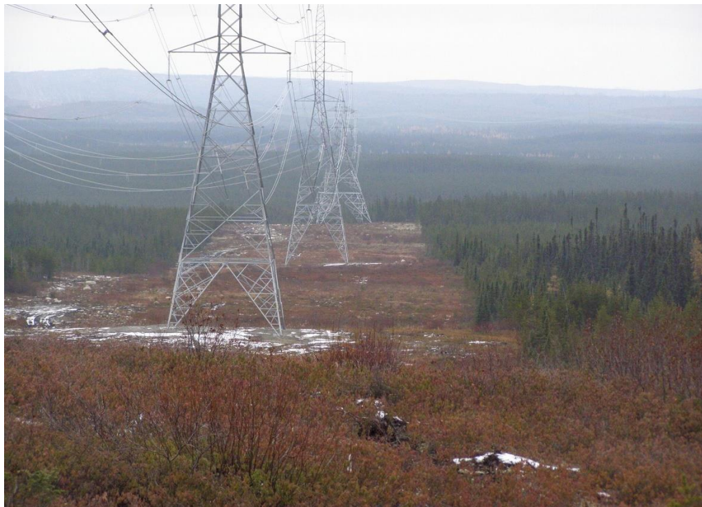
Figure 6 - Power line at Rose Site
