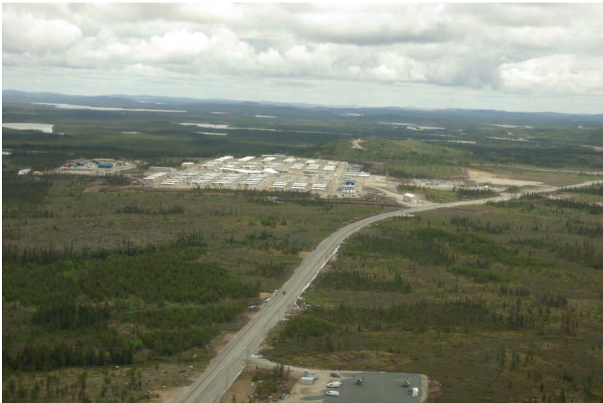
View of Hydro-Québec Rupert Camp and access road
